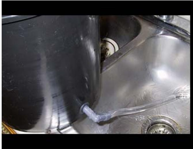
Start to assemble your Drip Ring. This will be above the hydroponics media and drip solution down. I use the screw tight T for irrigation, you can use barbed T's.
