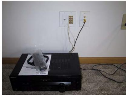
The CL2 wiring (3 conductor for R & L signal) was ran to our location and connected to the inwall RCA connector to simplify connection to stereo system aux input.
